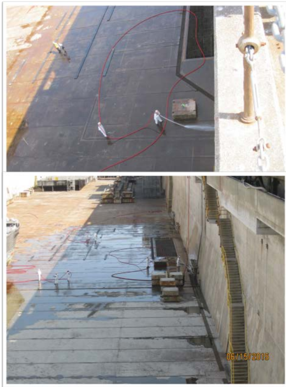
Figure 58. Photos of dry dock cleaning after dry dock dewatering.
